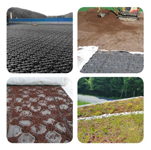
The roof garden panels are connected through special clips, which give stability and ability to adapt even on curved surfaces.
